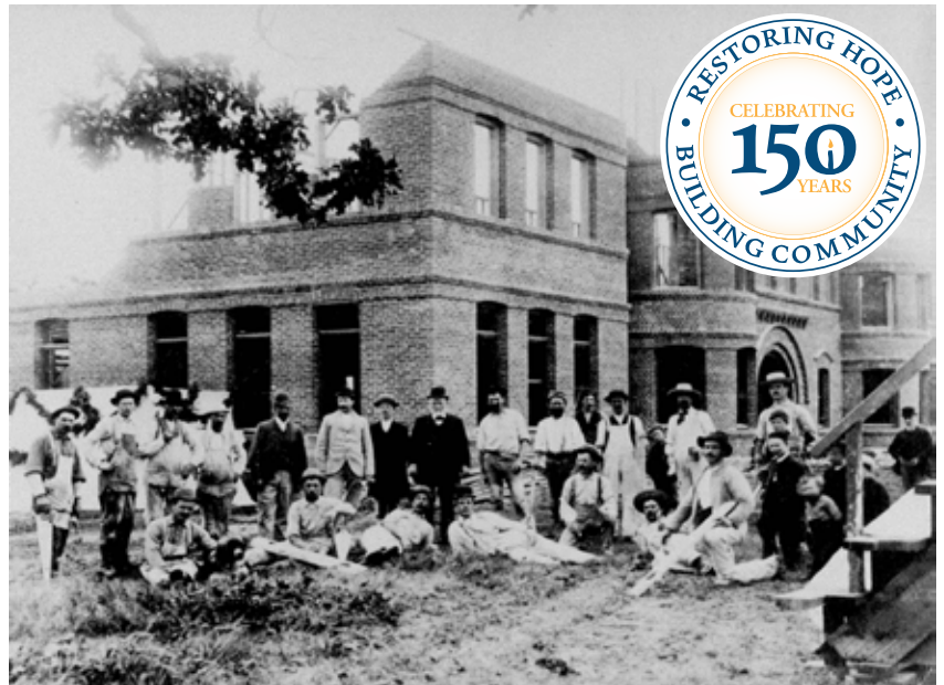
CONSTRUCTION OF THE TAYLOR BUILDING, JULY 1892
