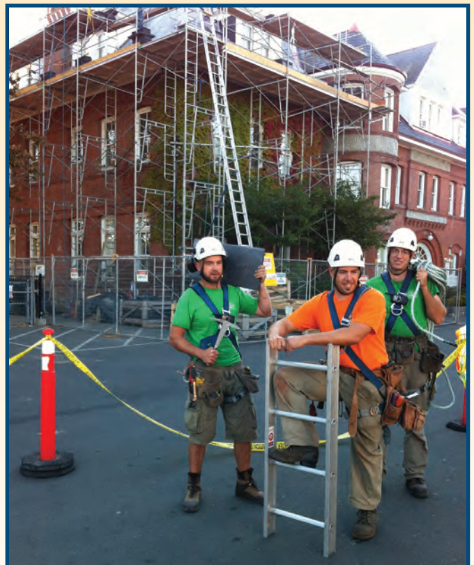
The Grist Team begins work on The Taylor Building
